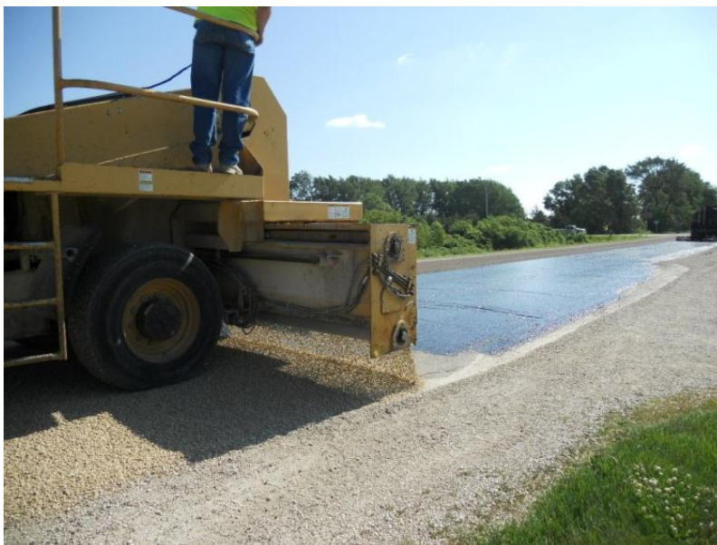
Figure 5: Chip Seal Application (photo taken by author)
