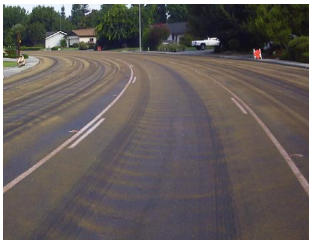
Figure 39: Fog Seal with Sand (Brownridge and Fox 2011)
