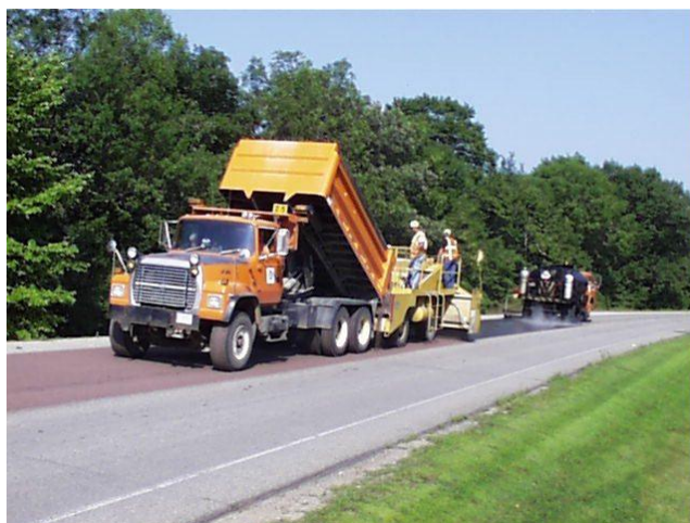
Figure 7: Asphalt Distributor Followed by Chip Spreader (photo taken by Cliff Plymesser)
