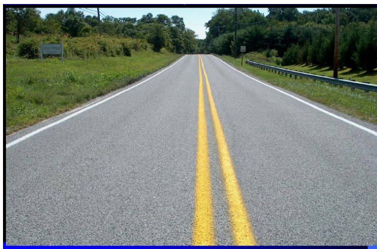
Figure 29: Good Chip Seal Result (Rizzuto 2008)
