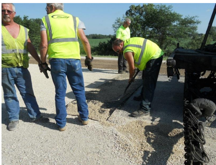
Figure 26: Application End on Mat (photo taken by author)
