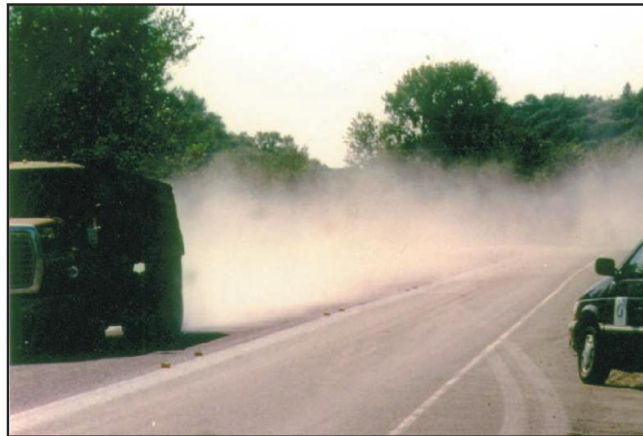
Figure 30: Dusty Aggregate Chip Seal (Wood et. al. 2006)
