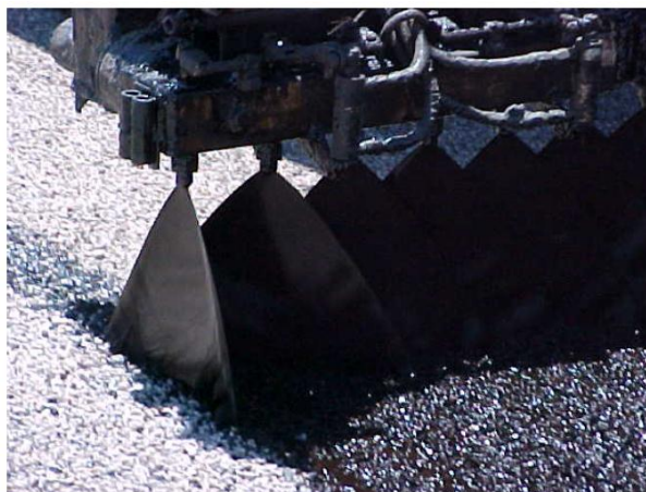
Figure 40: Inappropriate Nozzle Angle Alignment (MTAG 2007)
