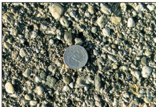
Figure 13: Well Graded Chip Seal Application (Wood et. al. 2006)
