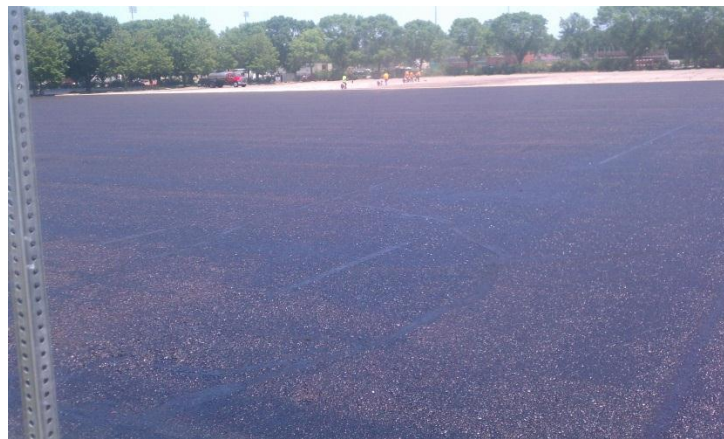
Figure 38: Fog Seal on Parking Lot (photo taken by author)
