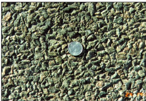
Figure 12: One-sized Chip Seal Application (Wood et. al. 2006)
